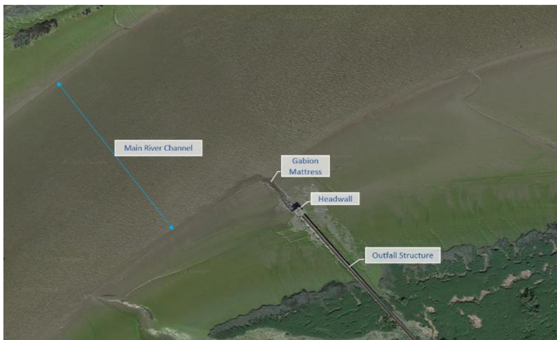
FIGURE 16-21: OVERVIEW OF OUTFALL STRUCTURE
